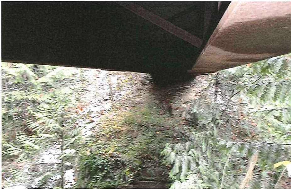
CK-2041 Abutment Right Bank
