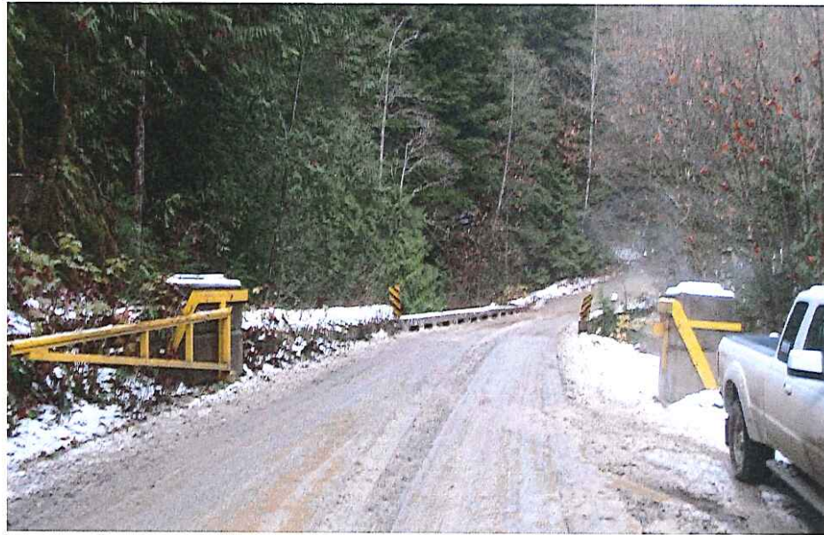
CK-2041 Approach Right Bank
