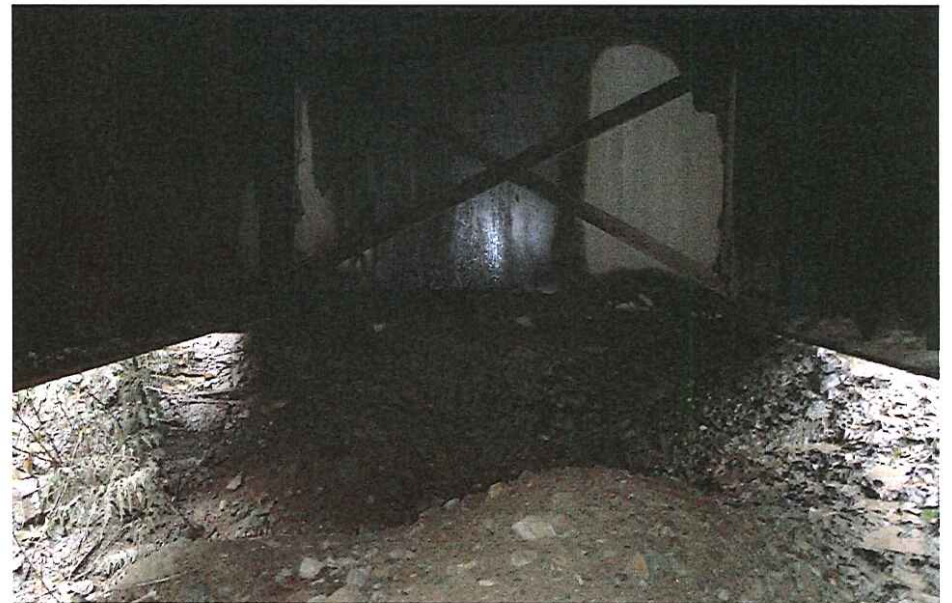
CK-2041 Abutment Left Bank
