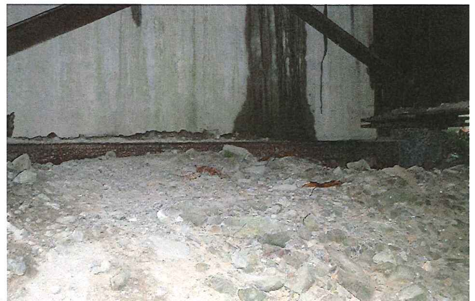
CK-2041 Abutment Right Bank #2
